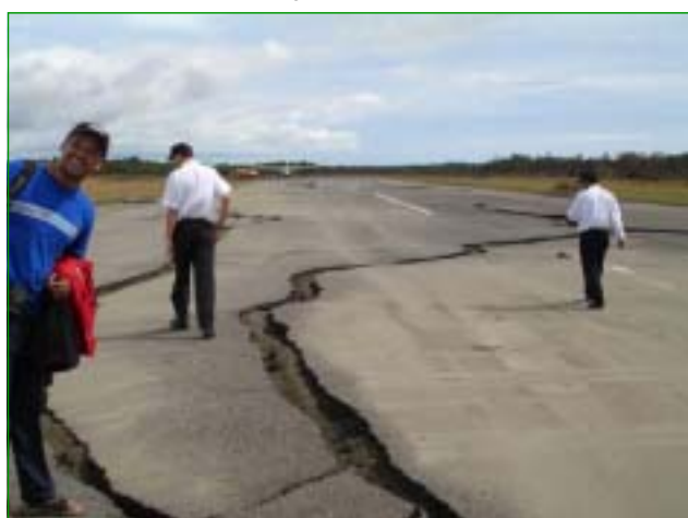
An earthquake cracked runway requires pilots to exercise slalom skills on take off and landing
