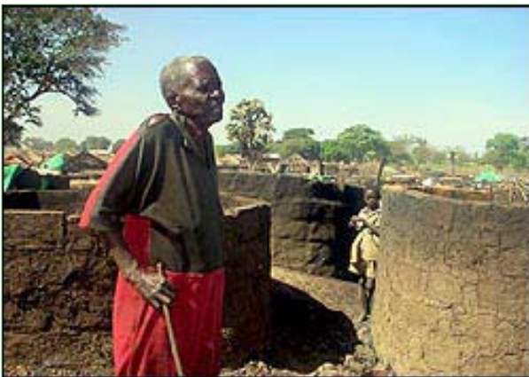
Ugandan refugee camp constructed of baked mud (the only available building material) - note the lack of roof cover
