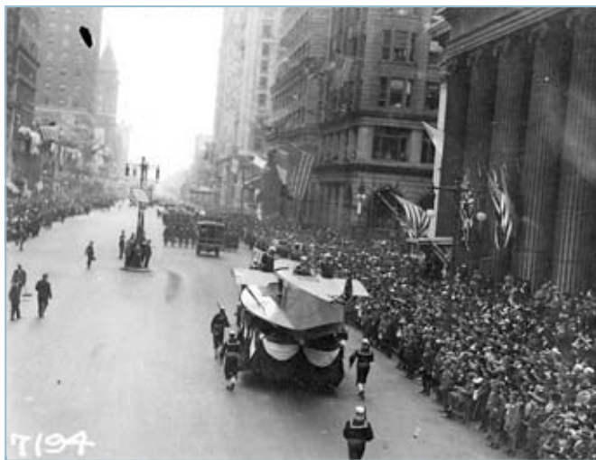
Liberty Loan Parade at Philadelphia, 28 September 1918 Naval Aircraft Factory float, featuring the hull of a patrol seaplane, going south on Broad Street, escorted by Sailors with rifles.
