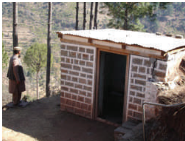
A recently installed permanent latrine in Kamra, northern Punjab province
